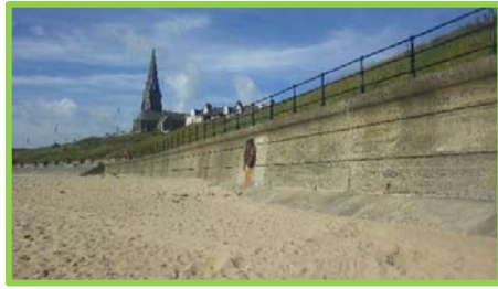
Concrete wall in good condition (/4701c17).
