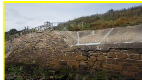
Concrete repairs, gaps in joints of stone wall (/4801c05).
