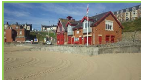
Concrete protection to Lifeboat Station in good condition (/4701c08).
