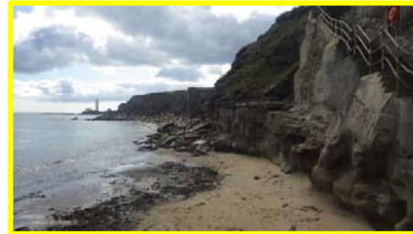
Evidence of minor rock falls and slips between Hartley Cove and Curry's Point (/4401c23).
