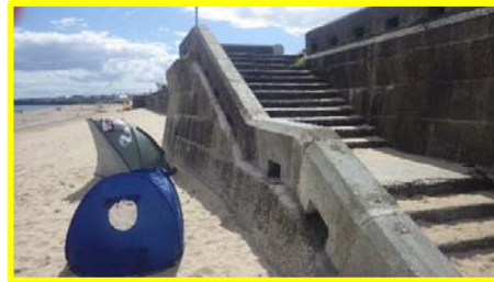
Steps in good condition, repairs carried out to joints (/4501c07).
