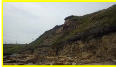
Evidence of slippage and rock fall around Sharpness Point (/4701c26).
