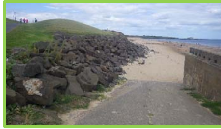
Revetment Briardene in good condition, sand levels good (/4501c06).
