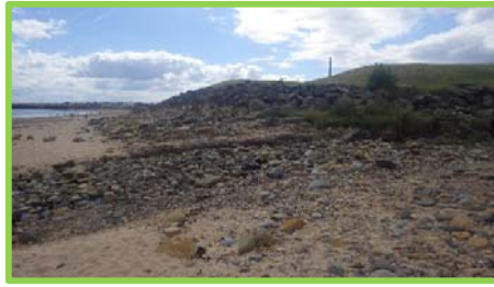
Revetment Briardene in good condition (/4501c06).
