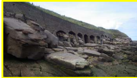
Arched retaining wall at Freestone Point (/4801c04).
