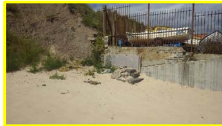
Repairs to south end of boatyard in good condition, high sand levels (/4501c05).
