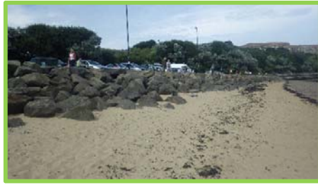
Stone protection in good condition (/4801c09).
