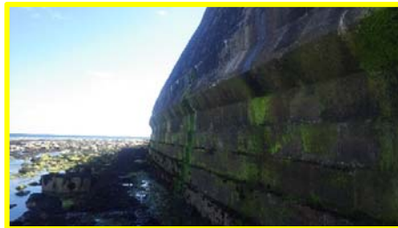
Wall in fair condition, minor repairs to joints required (/4601c06).
