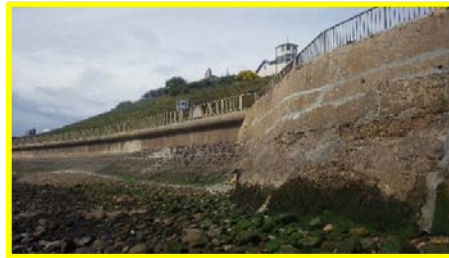
Repairs to concrete cracks (/4801c06).
