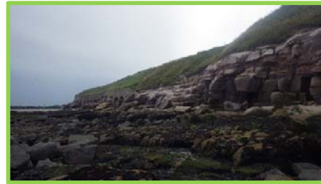
Fractured rock at Freestone Point (/4801c11).
