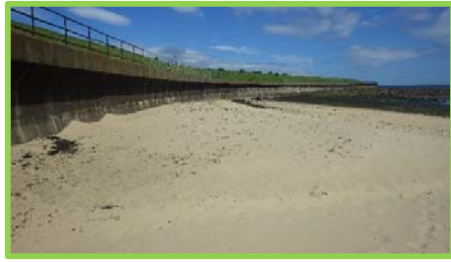
Trinity Road seawall in good condition, sand level good (/4501c04).
