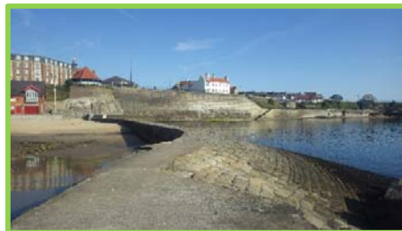
Cullercoats North Pier in good condition following repair works (/4701c07).
