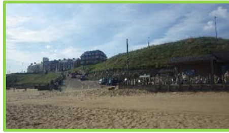
Timber and concrete protection to Crusoes Café (/4701c22).
