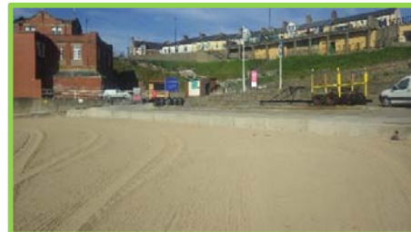
Concrete protection to steps in good condition. Sand level good (/4701c08).
