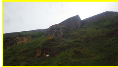
Evidence of slippage down from Tynemouth Castle (/4701c30).
