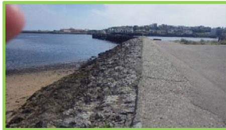
Pitched stone to jetty in good condition (/4801c10).
