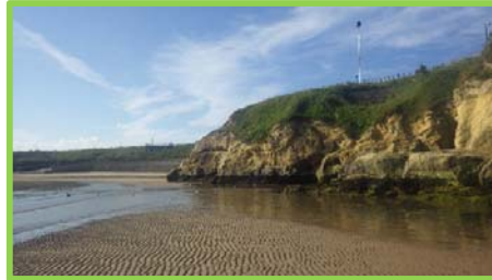
Cliffs centre of Cullercoats Bay in good condition, no evidence of rock falls (/4701c11).
