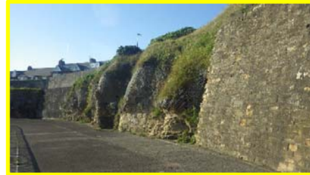
Rear wall well maintained, rock bolts and meshing (/4701c01).
