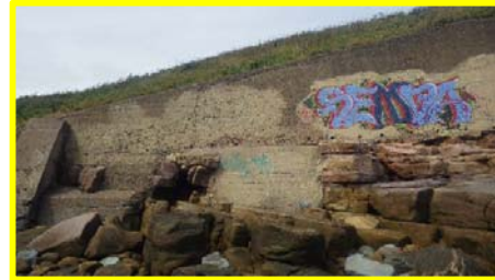
Joint of concrete wall and stone wall, fair condition (/4801c04).
