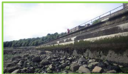
Previous patch repairs to vertical seawall in good condition (/4801c08).
