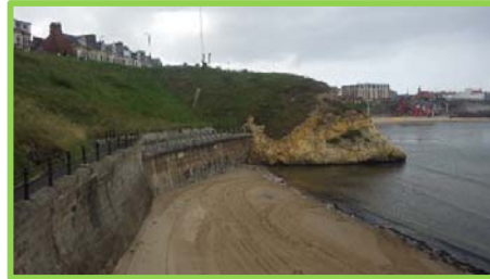
Cliffs centre of Cullercoats Bay in good condition, no evidence of rock falls (/4701c11).
