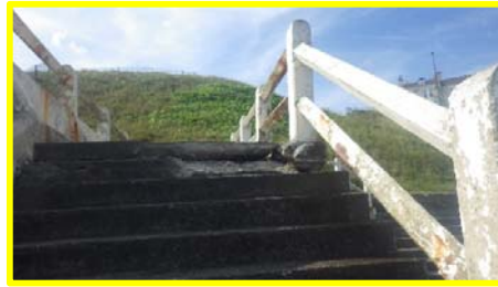
Damage to interior steps in pool (/4701c24).
