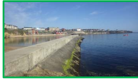
South Pier in very good condition following reconstruction, seaward side (/4701c15).
