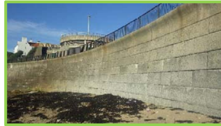
Wall in good condition, minor joint repairs required (/4701c05).
