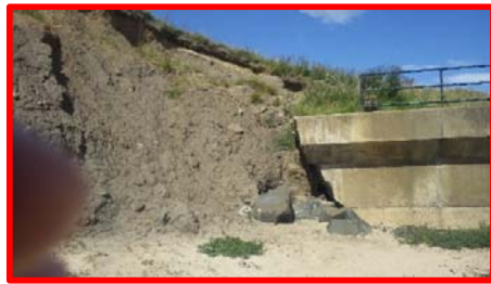
Outflanking at south end of wall similar to 2012 (/4501c05).
