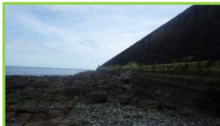
Tynemouth Pier, north side (/4801c01).
