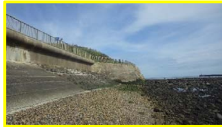
Masonry wall with concrete render adjacent to pitched stone revetment (/4801c06).
