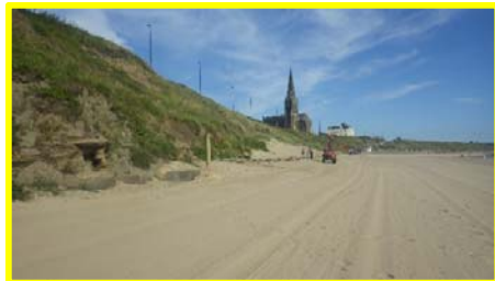
Erosion of Longsands dunes, remedial fencing and replanting underway (/4701c21).
