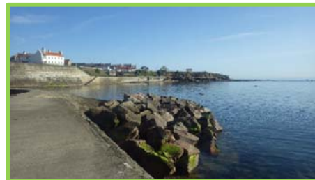
Stone protection in good condition North Pier (/4701c07).
