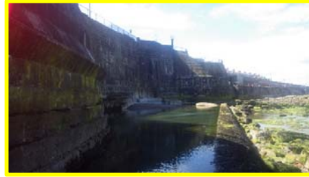
Hand railings appear in good condition (/4601c04).
