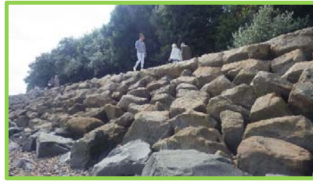
Stone protection in good condition (/4801c09).
