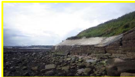
Concrete repairs to revetment (/4801c05).
